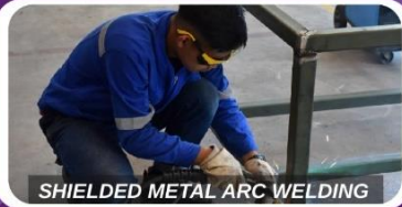
SHIELDED METAL ARC WELDING
